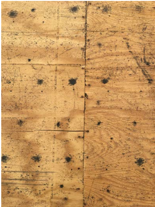
Plywood Sheathing, 8D Nail, 6" Spacing
