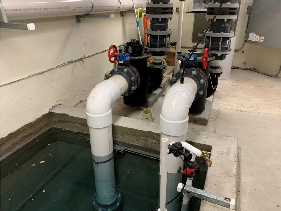
New Circulation Pumps and Pit
