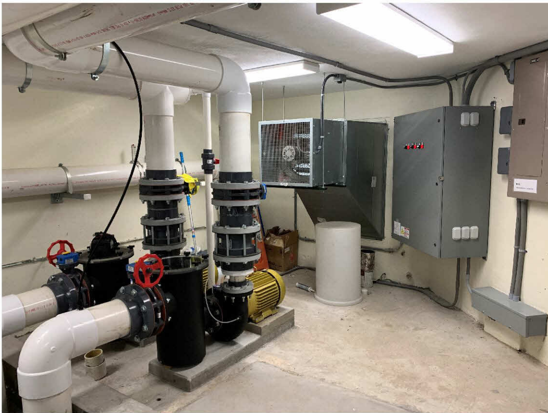
Circulation Pumps and Control Panel
