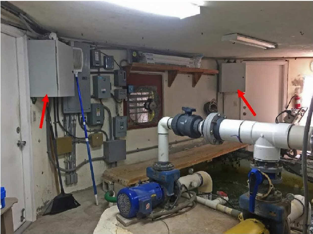
Circulation Pumps and Control Panel
