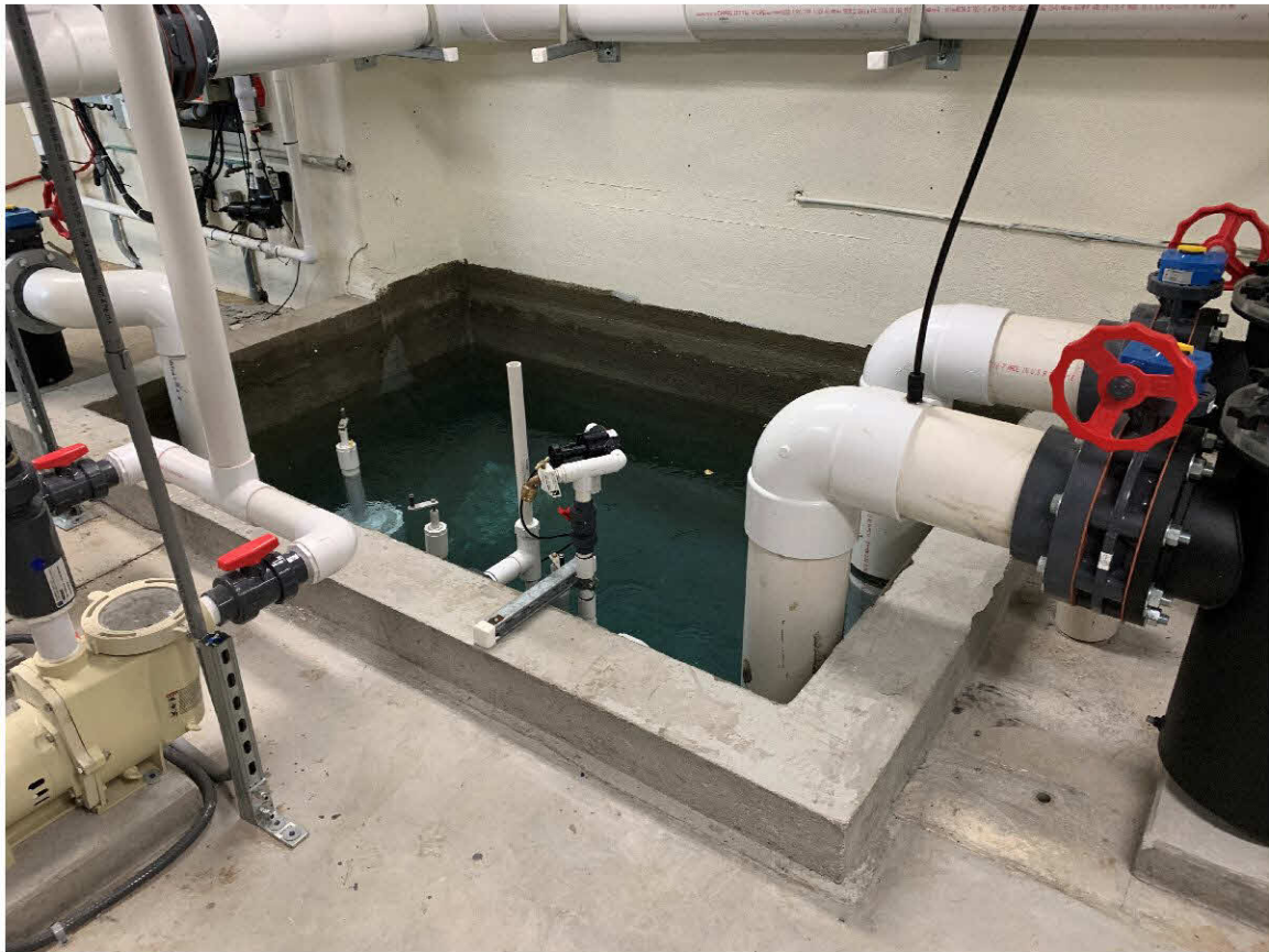
Sump with circulation intakes and auto-fill
